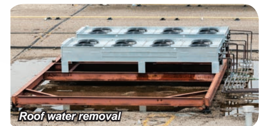
Vac out before patching
