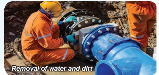
Removal of water and debris
