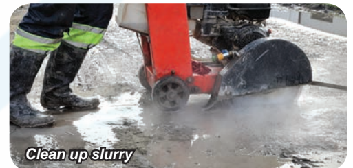
Removal of water and dirt
